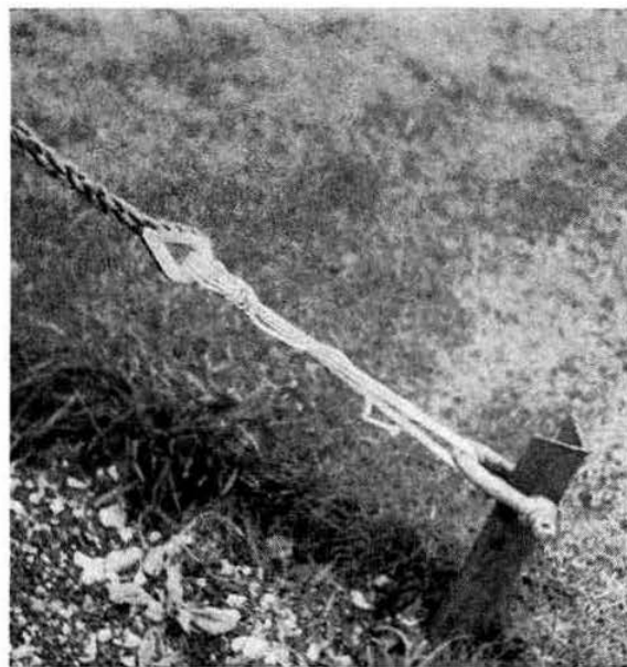
Alternative method of securing a guy to an angle-iron picket by means of a lanyard and large shackle
